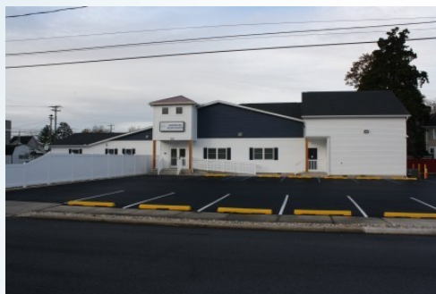
Newly Remodeled and Expanded Center
